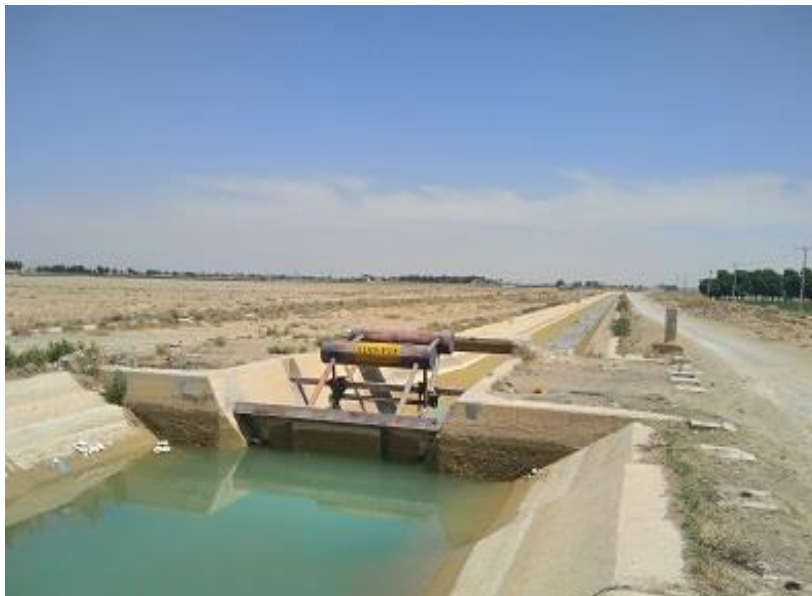
Fig.4. A valve divides the water between South Baraan village and the downstream village. A guard is assigned in this area to take care of the water distribution. Water theft from the village occurs when someone secretly opens the valve and redirects the water to the downstream village. Source: field observations
